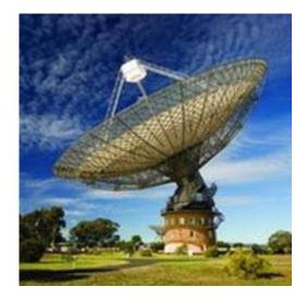
ability to detect weak radio signals from the cosmos at frequencies from 700 MHz to 1.9 GHz.
